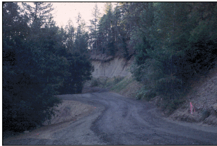
Figure 5-5. Outsloping Reduces Concentrated Flow on Road Surface
