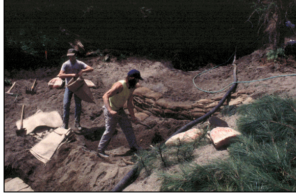
Figure 3-6. Grade Stabilization Structures are Incorporated into most Road-Crossing Excavations
