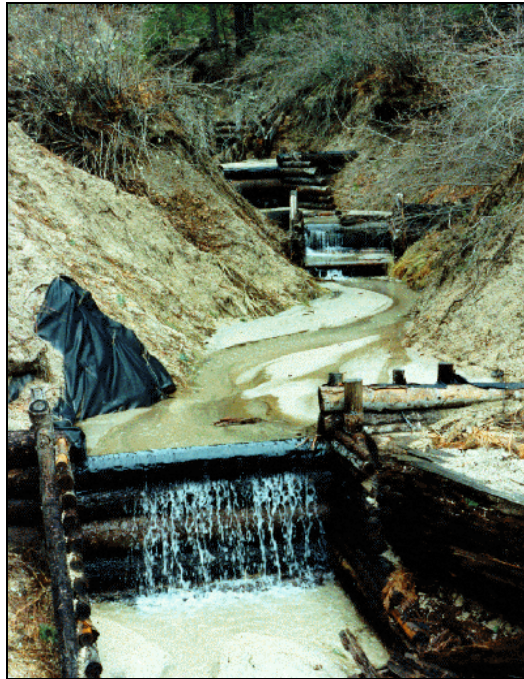
Figure 3-1. Log Grade-Stabilization Structure
