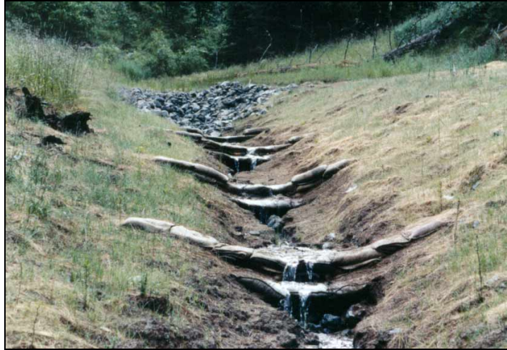
Figure 3-2. Soil/Cement Grade Stabilization Structure.
