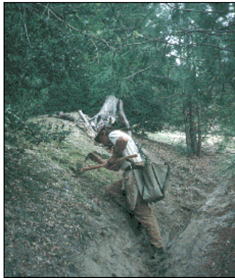
Figure 6-4. Planting to Stabilize Gully Banks
