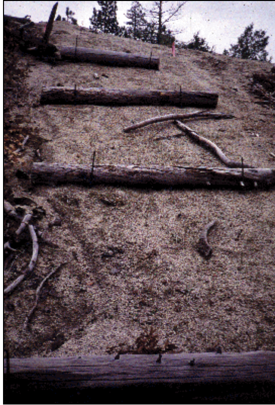
Figure 6-15. Cross Slope with Logs
