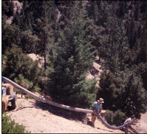
Figure 6-18. Using Straw Blower to Apply Mulch
