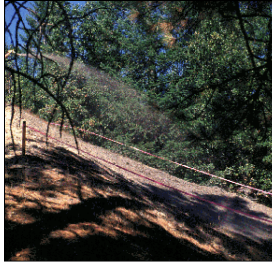
Figure 6-17. Lime-Based Tackifier Being Applied
