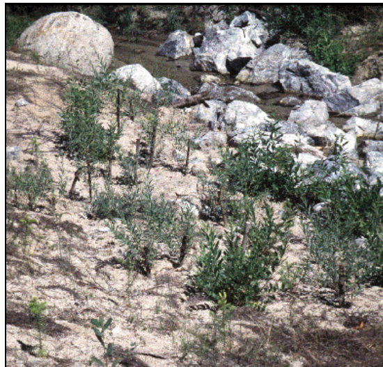
Figure 3-3. Willow Wattles and Willow Stakes in Channel
