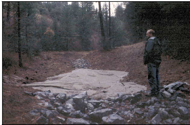
Figure 5-8. Excavated Sediment Traps Have Proven To Be Very Effective In GVC.
