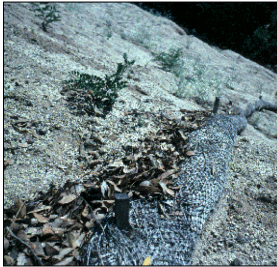
Figure 6-14. Straw Wattles Collecting Debris.
