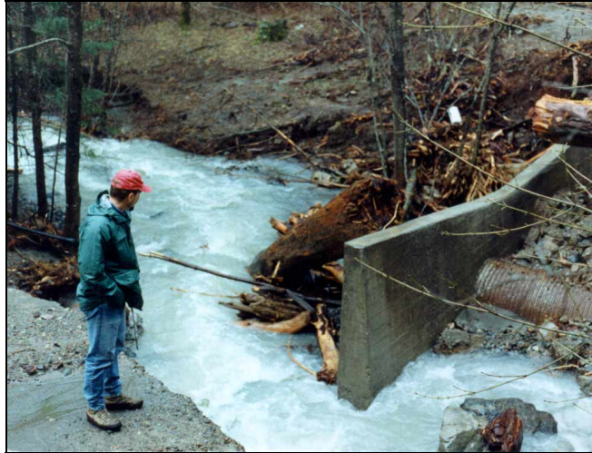
Figure 5-7. Culverts Will Inevitably Plug With Debris. Critical Dips At Crossings Will Ensure That Flows Remain In Stream Channels.
