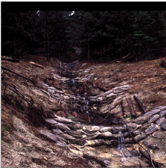
Figure 5-10. Soil/Cement Checkdam
