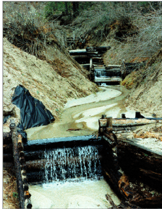
Figure 5-11. Log Checkdam
