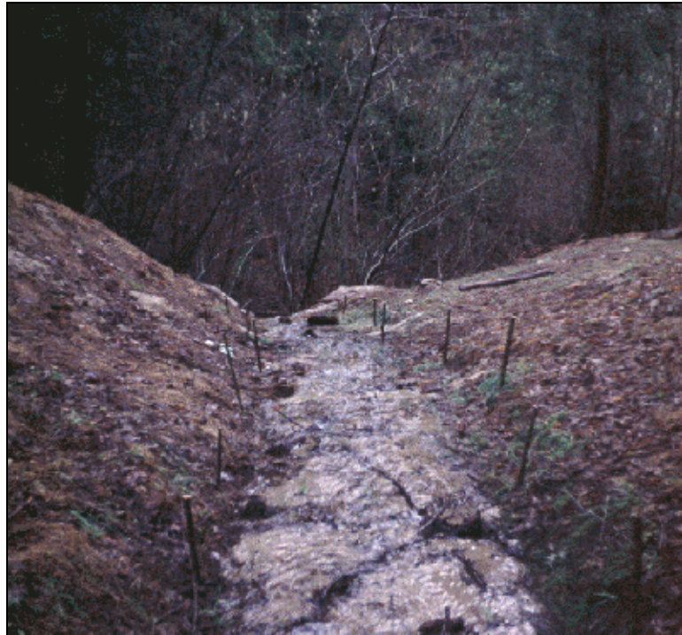
Figure 6-7. Willow Stakes Installed Along an Excavated Channel
