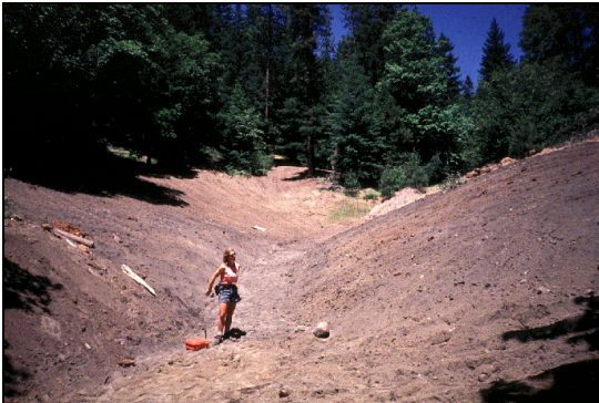
Figure 5-2. Unprotected Channel on 6/15/94.
