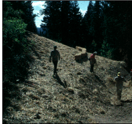
Figure 6-3. RCD and CCC Crews Spreading Mulch on Mechanically Treated Site.
