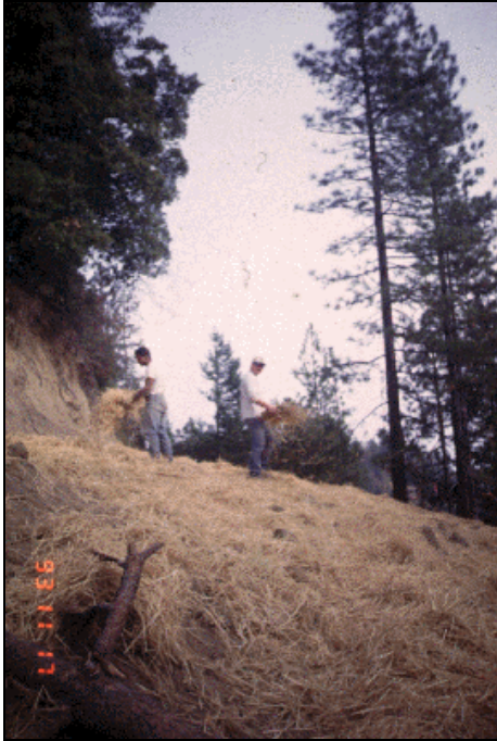
Figure 6-2. RCD Crew Spreading Mulch
