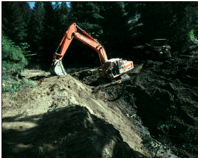
Figure 3-4. Heavy Equipment Removing a Road Crossing.
