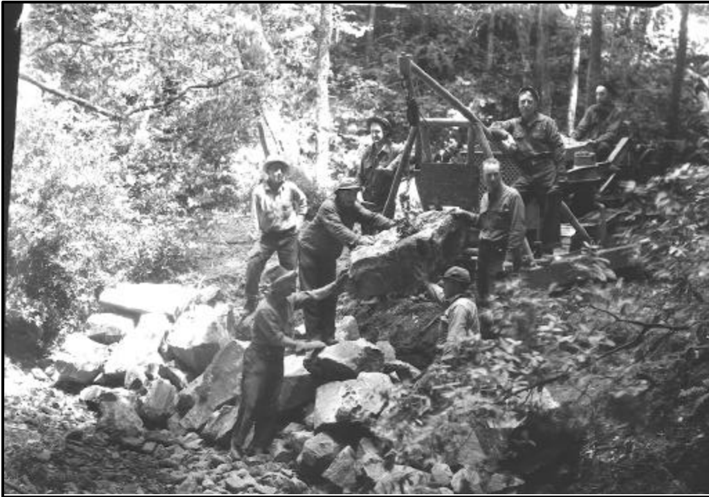
Figure 8. CCC workers placing large boulders on Redwood Creek in Muir Woods ca. 1934 (from NPS Archives).
