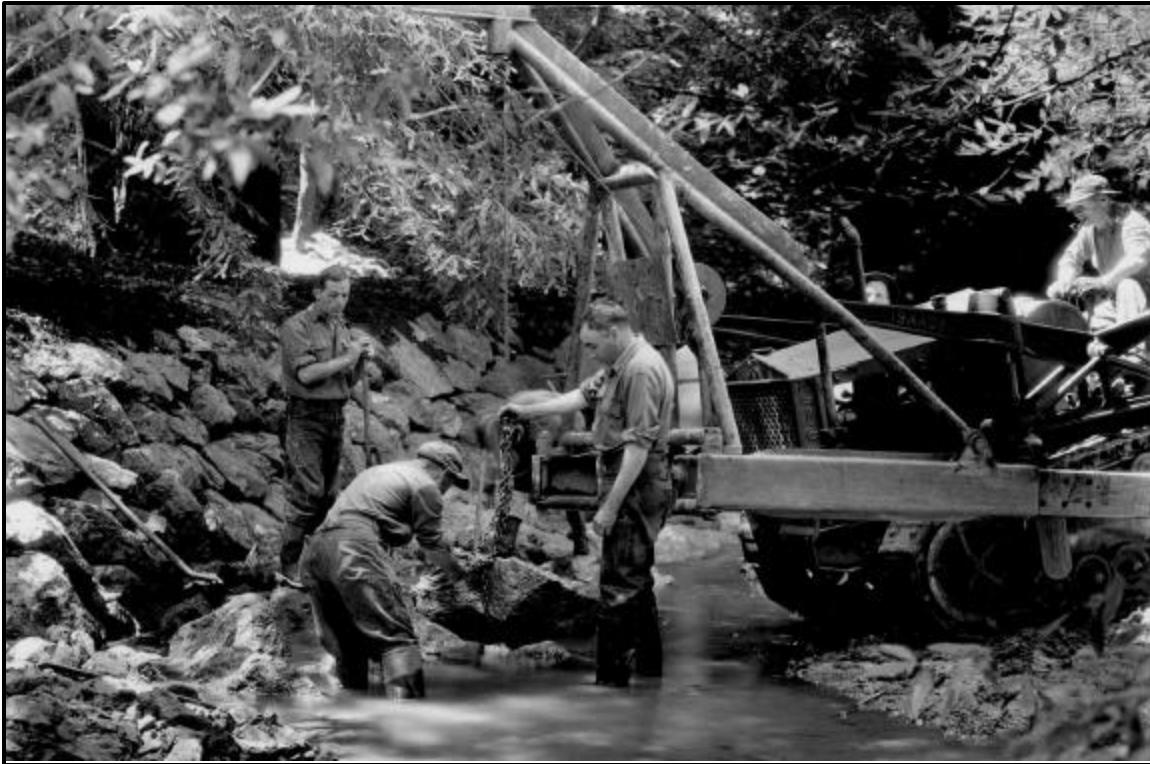
Figure 11. CCC workers with equipment in the streambed placing rock ca. 1936 (from NPS Archives).
