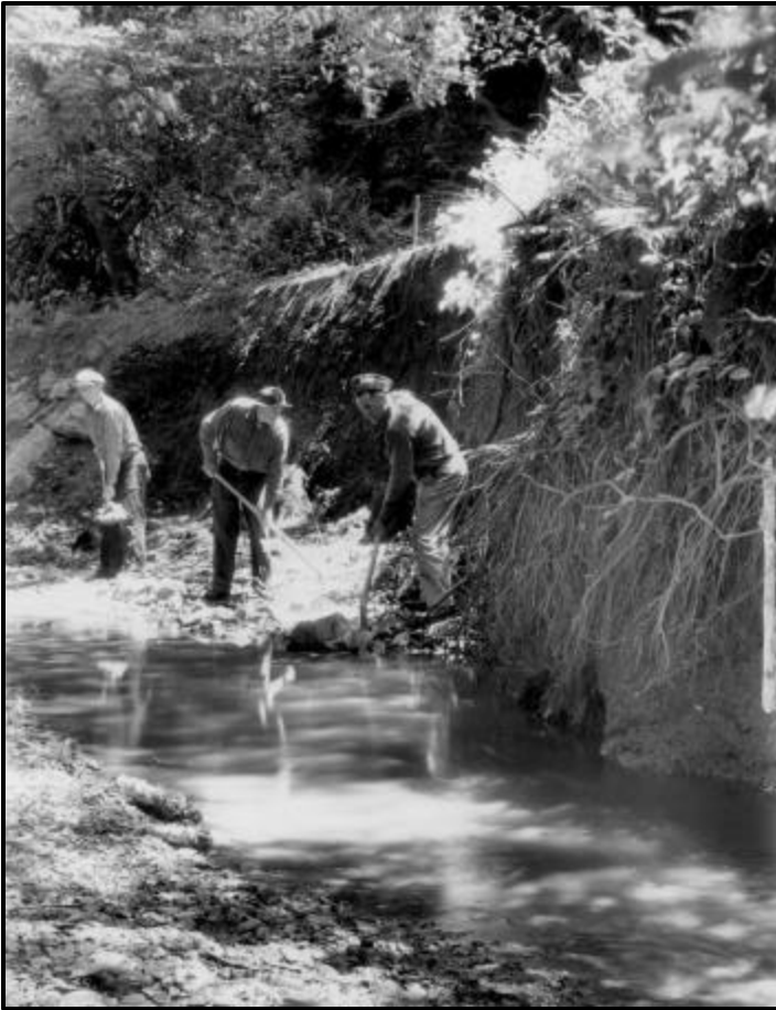
Figure 6. CCC workers in the Redwood Creek channel. Note the height of the bank in relation to the men and the roots exposed from scour (from NPS Archives).
