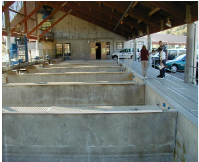
Don Clausen Fish Hatchery Facility at Warm Springs Dam, Sonoma County, California
