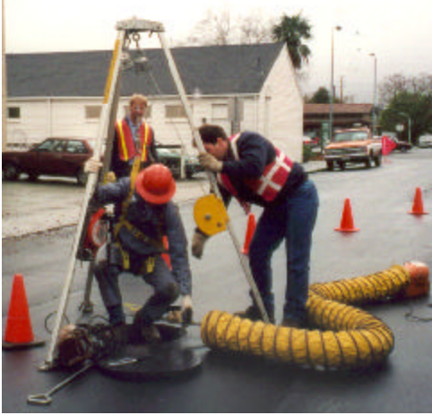
Staff receive ongoing training in spill response and pollution prevention
