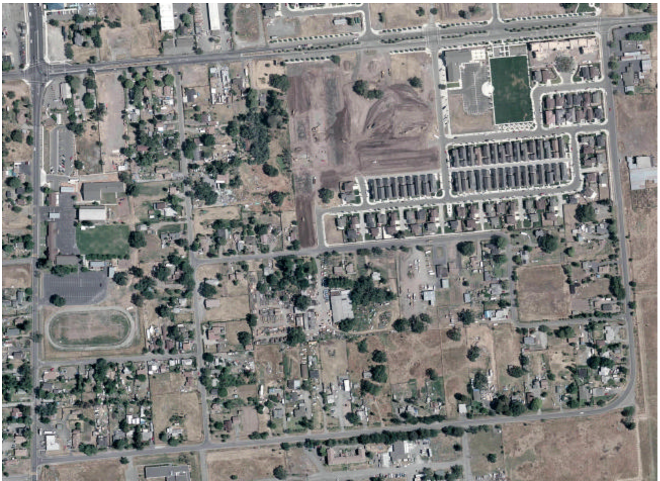
Aerial view of the Leddy Park area of Santa Rosa
