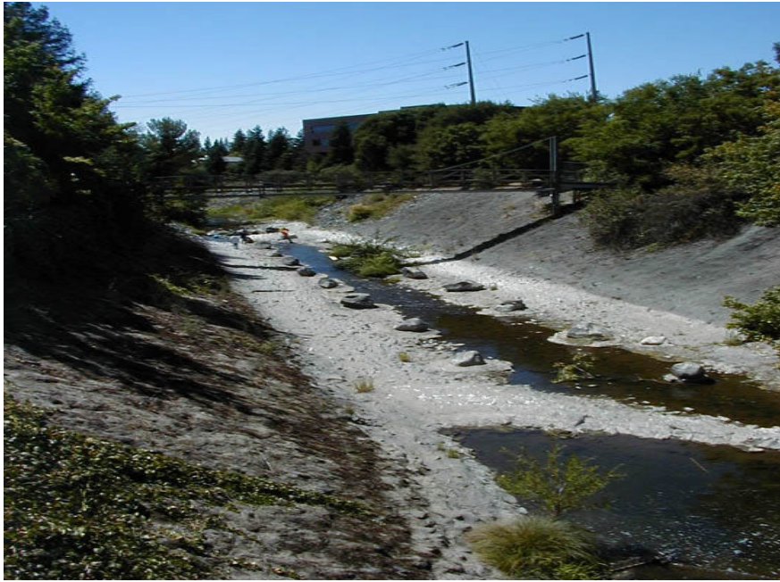
Santa Rosa Creek Prince Memorial Greenway - Phase IV prior to construction
