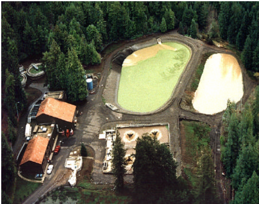
Aerial view of the Russian River County Sanitation District's wastewater treatment facility.
