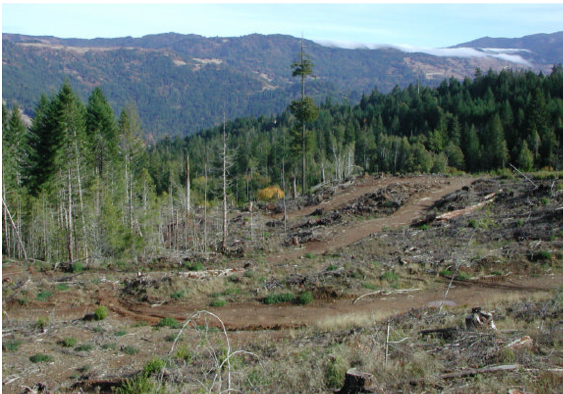
Figure 14. Recent clear cut in Redwood Creek watershed showing extensive tractor skid trails or temporary haul roads, which are not considered part of the road network but do add to changes in hydrologic function.
