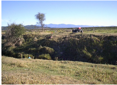
Middle cross-section - right bank facing southeast (9/01)
