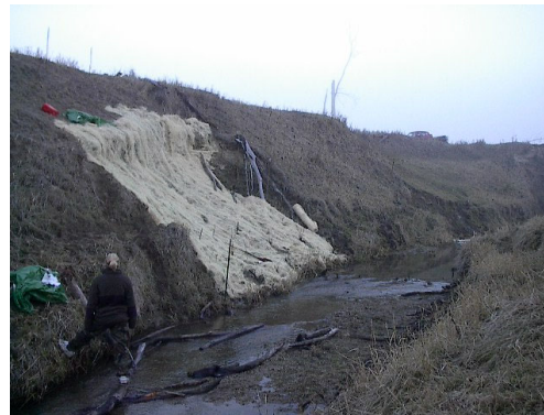
Bank with poplar matting in place
