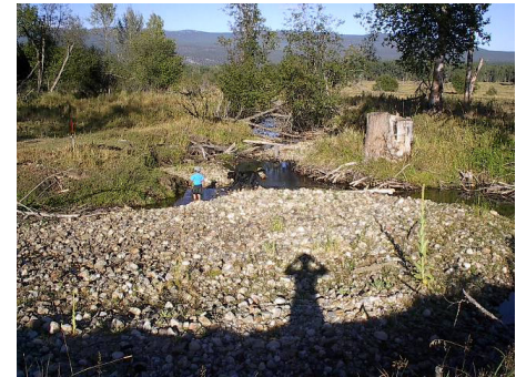
Upper cross-section - left back facing east (9/01)
