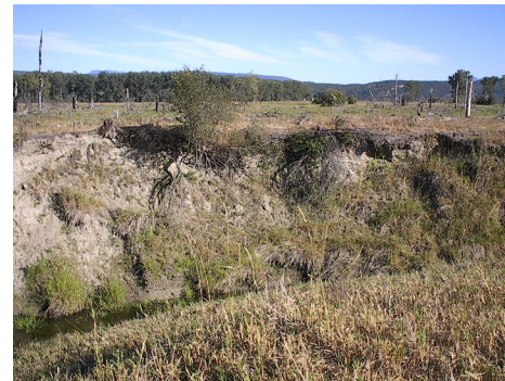
Primary cross-section - right bank facing east (9/01)
