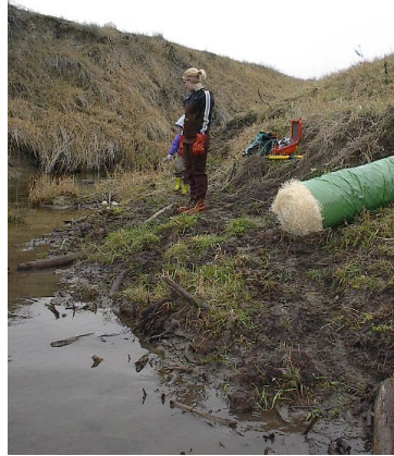
Unstable bank prior to placement of poplar matting
