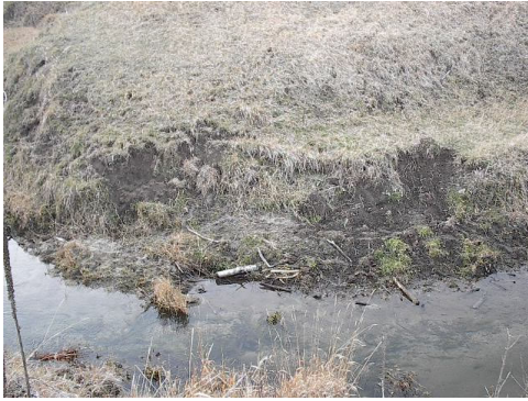
Unstable bank prior to placement of poplar matting
