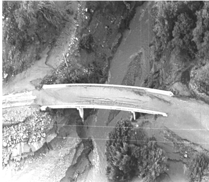
Figure 22 Slate Creek Bridge on Highway 96 Following the 1964 Flood.
