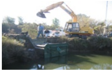
McBain and Trush recently completed construction of a 'fish friendly' tide gate allowing fish passage into Rocky Gulch.
