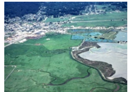
McDaniel Slough winding it's way through agricultural land near the mouth of Humboldt Bay. Photo courtesy of Mark Andre, City of Arcata
