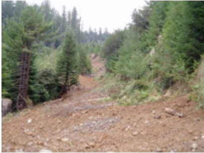
Headwaters Forest Reserve road decommissioning. Decommissioning old logging roads may help to reduce adverse CWE's caused by sediment.
