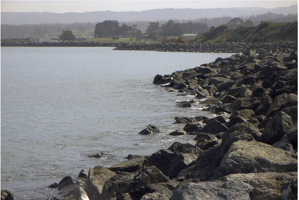
Figure 3. The shore of Entrance Bay of Humboldt Bay, Humboldt County, California is lined with rip-rap due to increased wave action. This photo was taken near the town of King Salmon, along the eastern shore of Entrance Bay.
