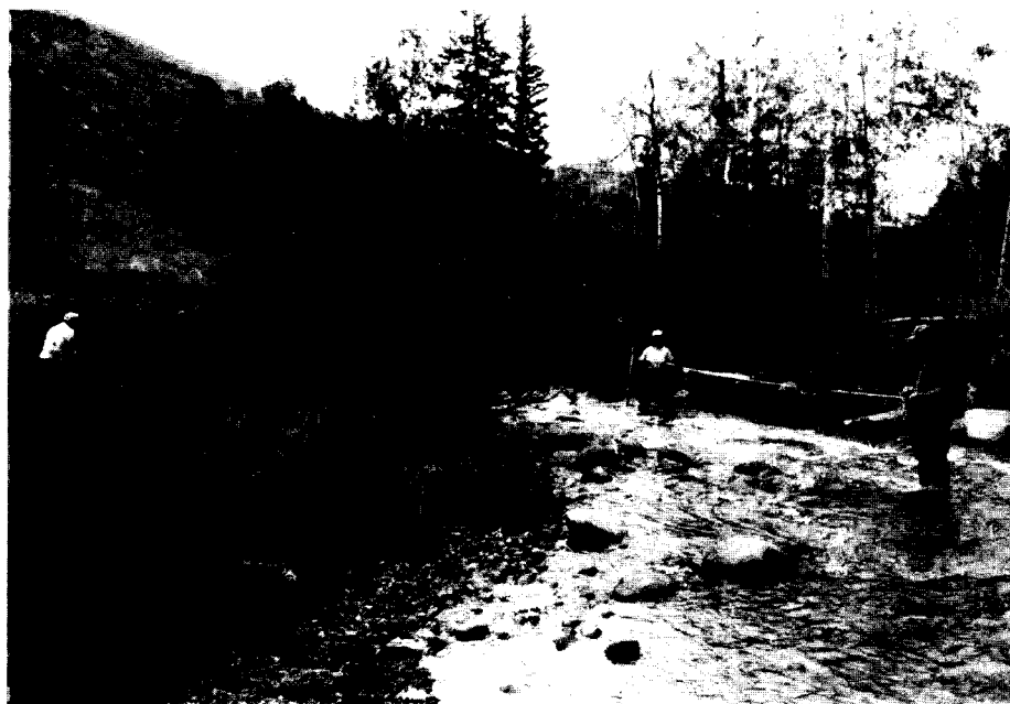
Figure 50. - Measuring along the channel centerline and staking.
