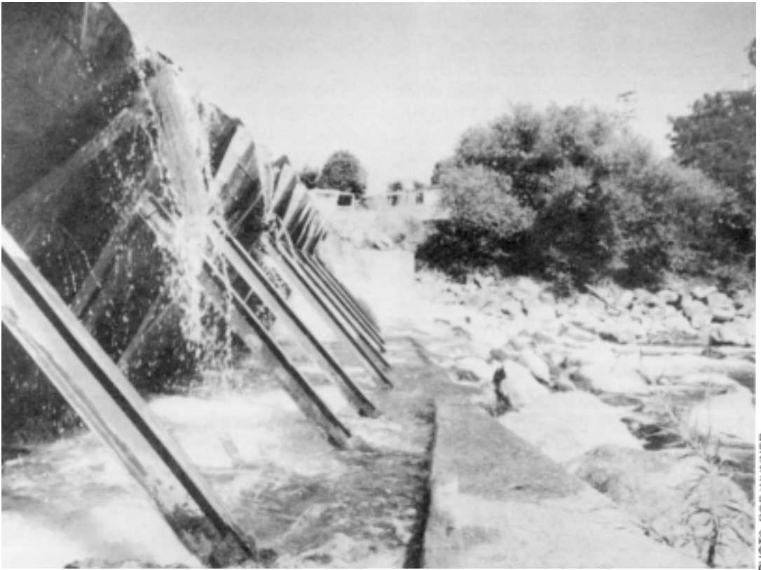
At Healdsburg, young salmon and steelhead are forced to plunge through the narrow opening in Sonoma County's dam, only to strike the concrete sill below
