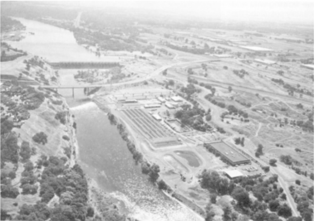
PHOTO: BUREAU OF RECLAMATION
