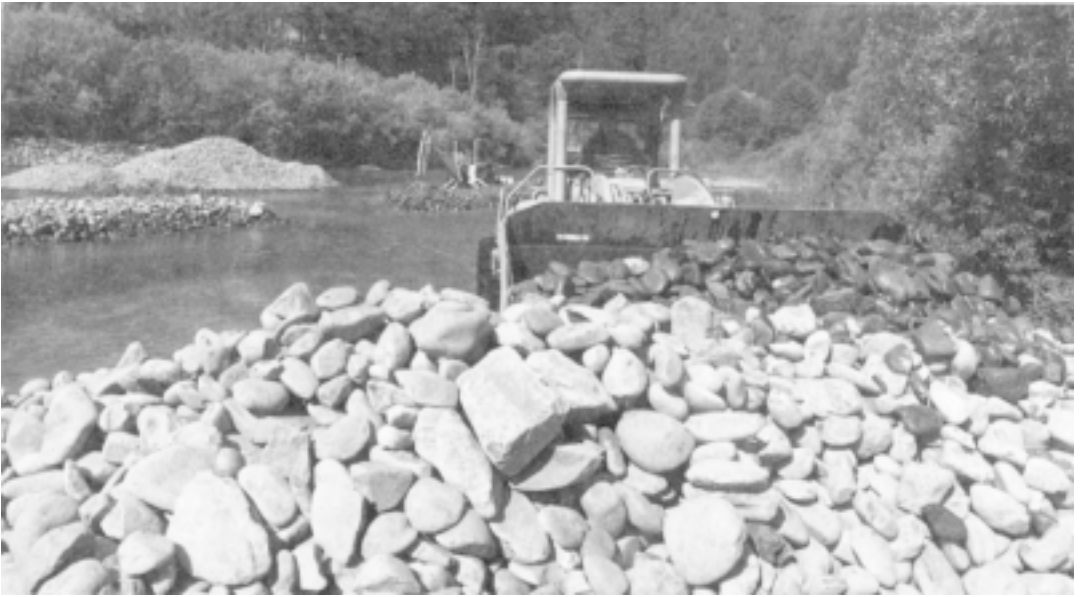
PHOTO: BUREAU OF RECLAMATION
